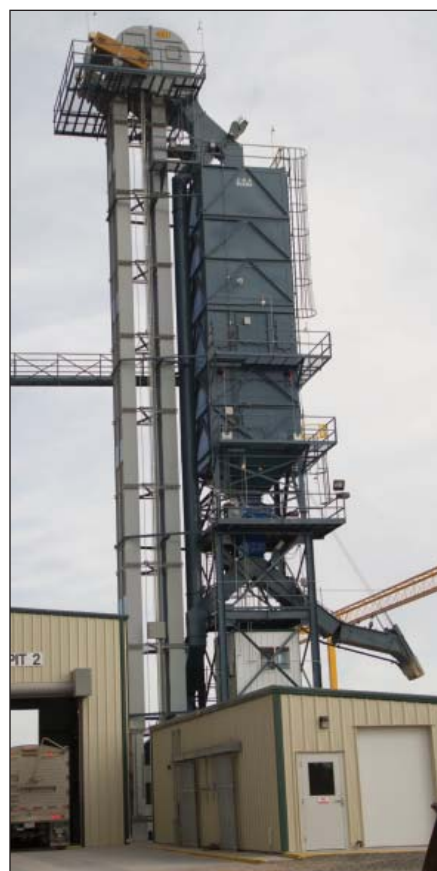
A C&A Scales bulk weigh scale with an extended upper garner for rail loadout. Photo by Alex Lord.
