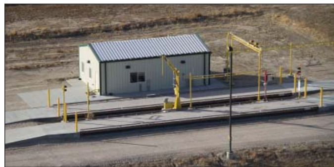
A separate scalehouse is equipped with two MidAmerica scales and Gamet probe. Photo by Alex Lord.
